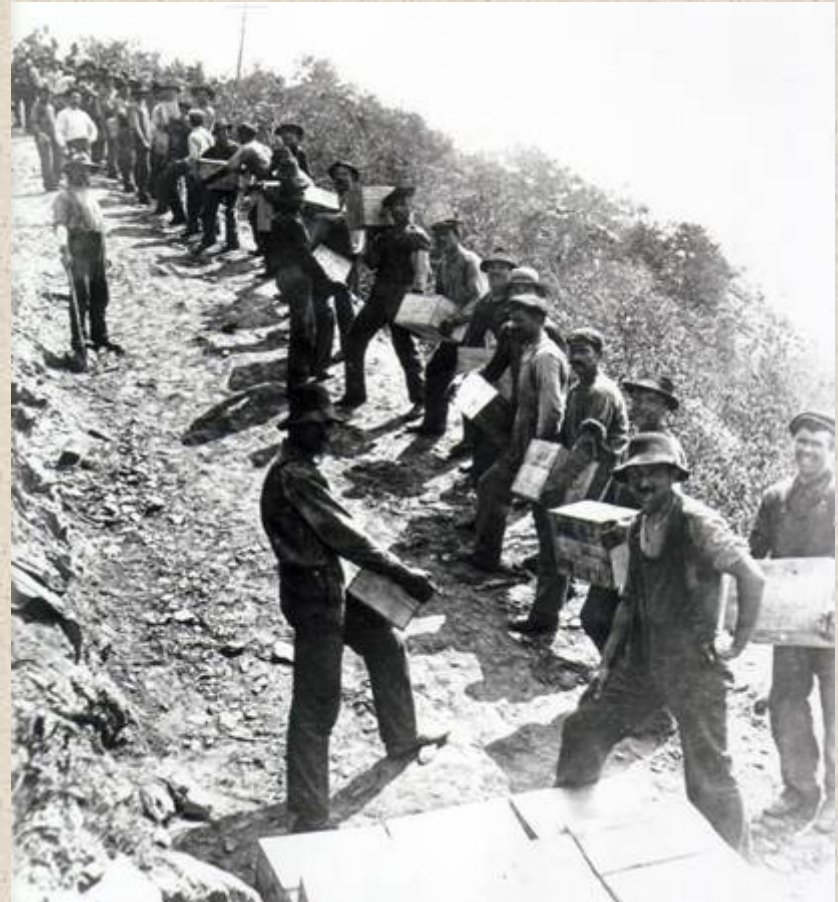
Rail workers moving dynamite during construction of the Pennsylvania Railroad, 1906
