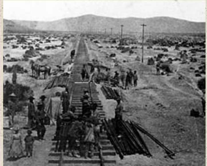
Central Pacific workers laying rail in Nevada
